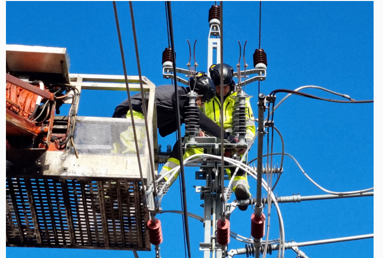
Installation of an open-air switchgear system from Hughes
